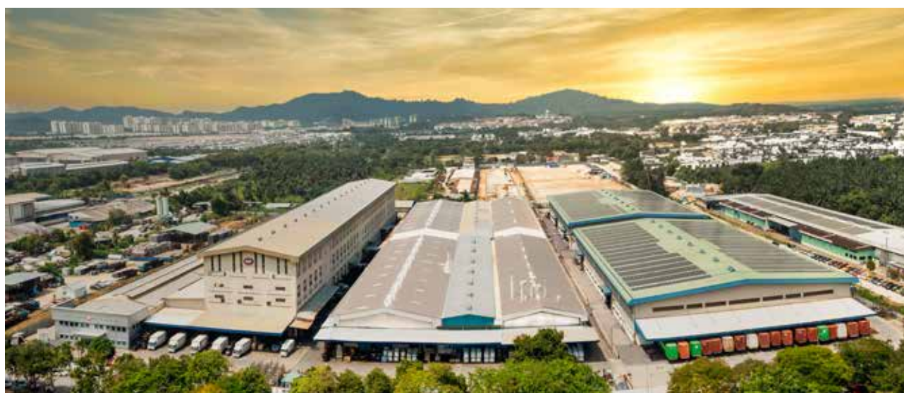
NHF's headquarters and manufacturing facilities in Klang, Selangor, with rooftop solar panels installed on one of the buildings.
